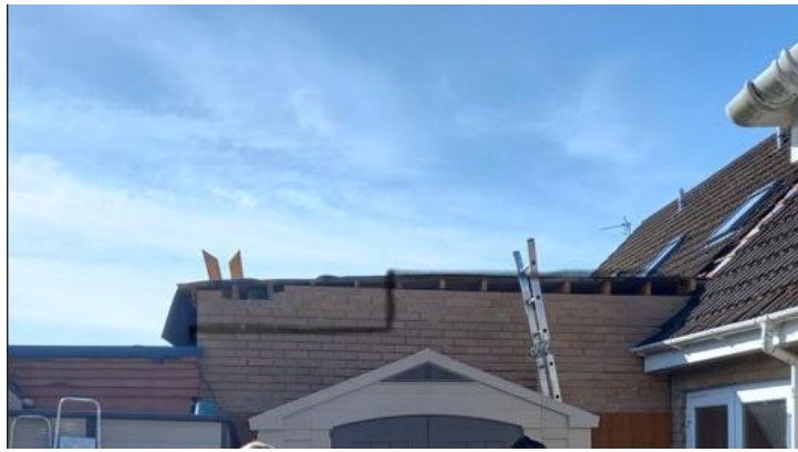
Fig. 6 – Relationship between the extension and 37, Hunters Ridge part way through construction
